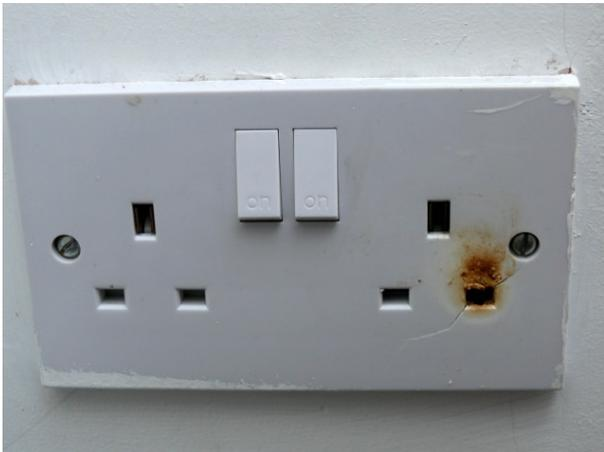
If you notice and heat or physical damage to sockets, stop using that socket and get a qualified electrician to investigate the problem.
